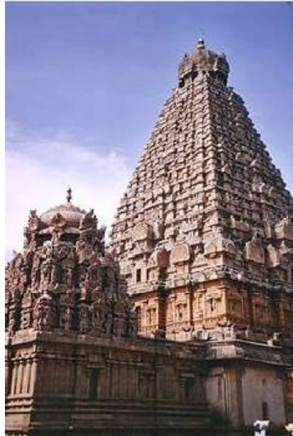
Fig. 5.2 Detail of the Main Gopura (Tower) of the Thanjavur Temple
